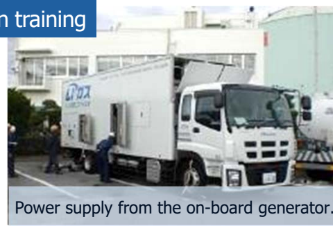
A mobile power generator car connected to power receiving equipment at the base.
