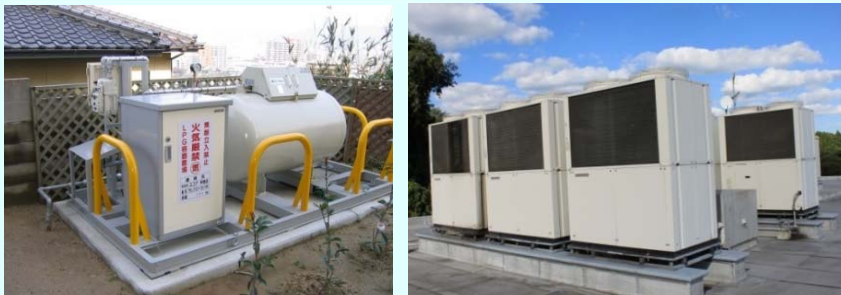
→ Installing bulk units and GHP at the shelters
