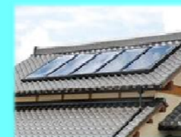
Solar water heater
