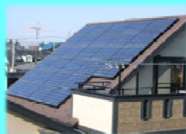
Photovoltaic electricity generation
